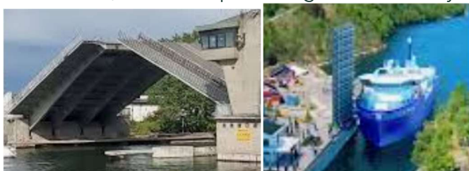
Figur 12. Prinsipp for vippebro
